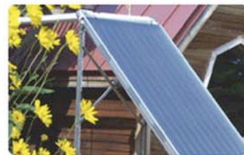
Location: Bethlehem, NH System: Hot water - flat plate collector
